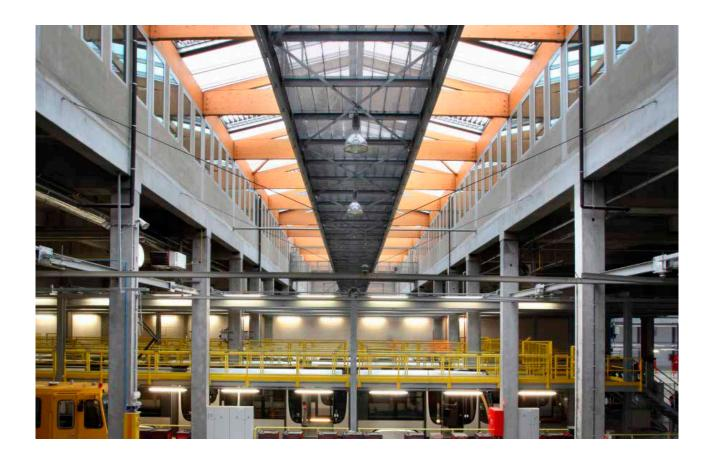
**PROJECT DESCRIPTION** Complete electrical installation of a new maintenance hall for trams. Supply and installation of a new MV cabinet, supply and mounting of the low voltage installation, including: GLVB, distribution panels, lighting, video surveillance, sound system, access control, fire detection, supply and installation of 750V DC contactors to power the overhead lines.
