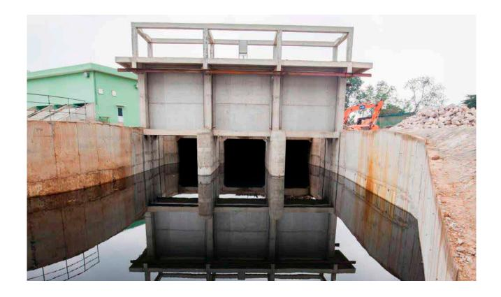
**PROJECT DESCRIPTION** Preparation of civil engineering guide plans, supply of 6 auger pumps with a capacity of 3m<sup>3</sup>/s each, 3 vertical pumps with a capacity of 3m<sup>3</sup>/s each, automated rough screening & fine screening (PS2), hydraulic valves & stop logs, lifting equipment, instrumentation, low voltage electrical panels, systems automation and monitoring, centralised remote control for the three pumping stations.
