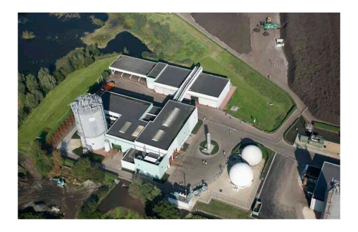
**PROJECT DESCRIPTION** Electrical composting installation according to the Dranco principle. Siemens PLC. Instrumentation (EEx and non EEx): temperature and level monitoring, flow meters, ultrasonic transducers. **UTILITIES** phone & data network, lighting, fire detection, video surveillance, tracing. **STUDY** electricity (boards & routing), instrumentation. **SCOPE OF WORKS** complete electrical installation, board manufacturing, support and commissioning.
